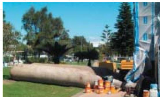
*EPA requirements on some repainting projects require full filtration of the extracted air.*
