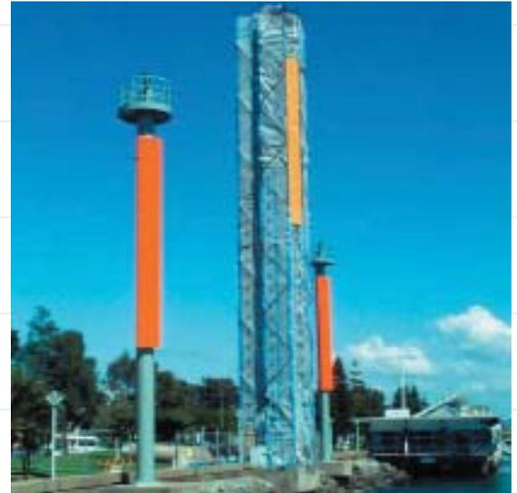
*Environmental controls are much more stringent where maintenance painting is required, even for non-hazardous coating. This navigation tower required full containment for its refurbishment.*
