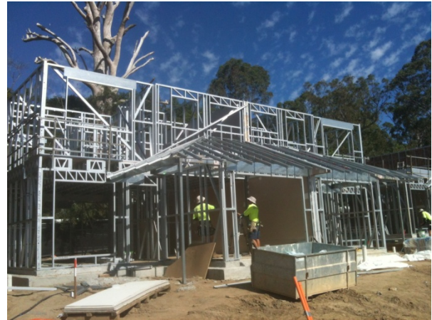
Photograph 3: Townhouses under construction
