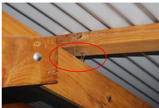
(a) batten to rafter connection
