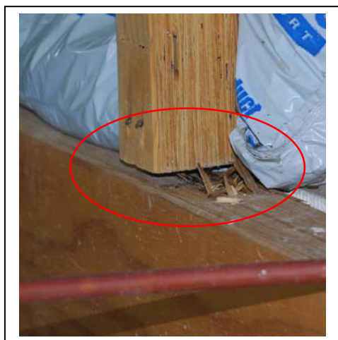
(b) connection at bottom of strut
