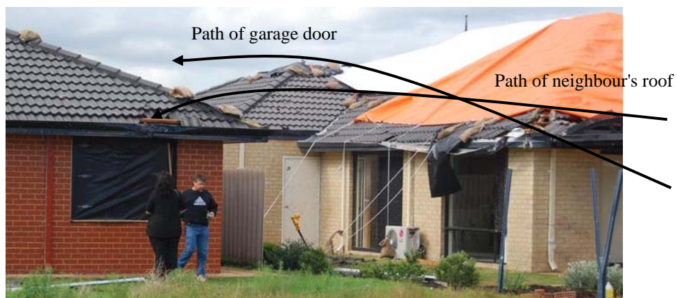
Figure 4.13 Debris damage to tiled roofs
