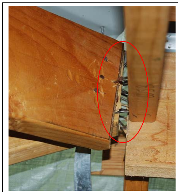
(c) connection at hip rafter
