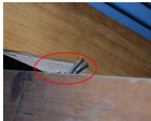
(b) rafter to top plate connection
