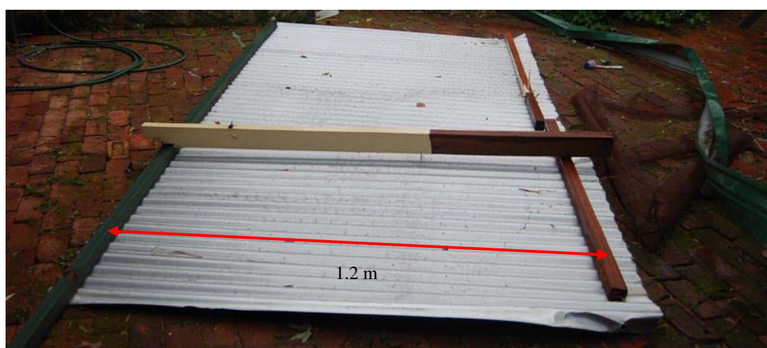
Figure 5.1 Batten spacing on verandah
