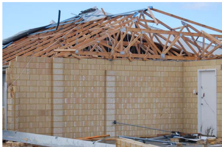
(a) roof batten loss
