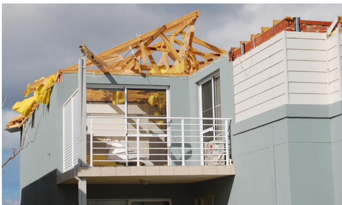
Figure 4.7 Loss of roof structure – two storey house
