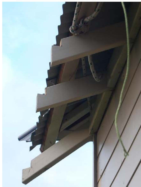
(b) lifted roof battens near corner of roof
