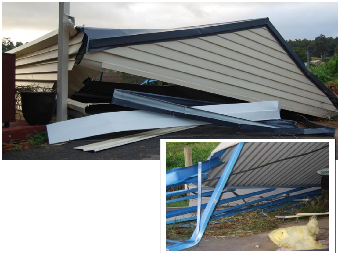
Figure 4.15 Racking failure of garage
