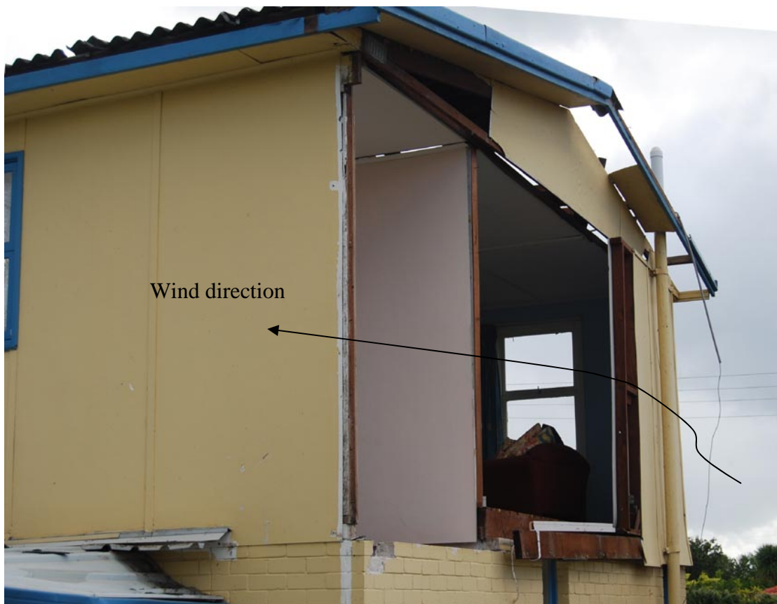
Figure 4.12 Loss of a side wall under combined internal pressure and external suction
