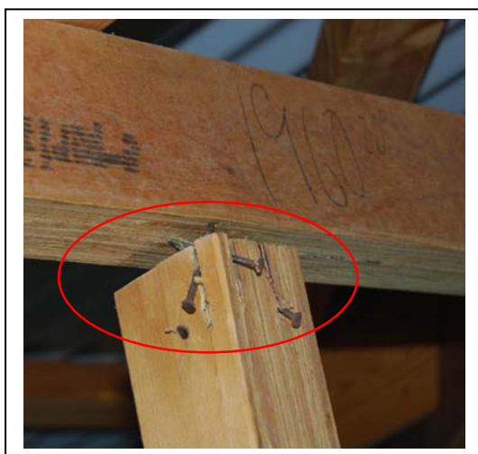
(a) connection at top of strut
