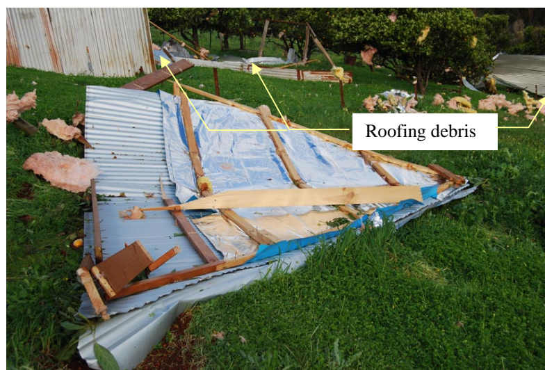
Figure 4.14 Debris strewn more than 50 metres from house
