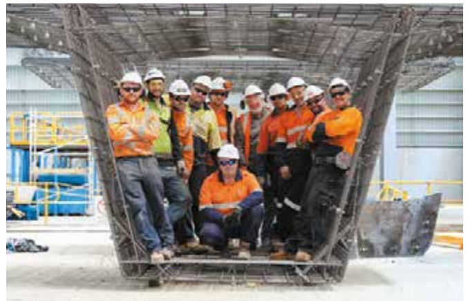
Workers inside a steel frame made for concrete segments
