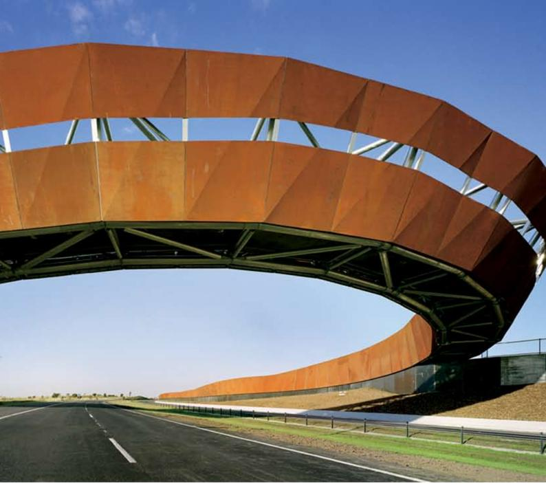
efficient shape. The steel structure weighs 70 tonnes supporting over 250 tonnes of bridge deck, superimposed dead and live loads.
