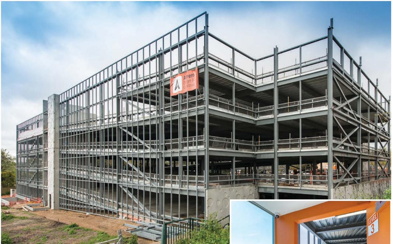
“Once primary steelwork reached level three, the next panel was erected followed by the secondary steel,” he said.
