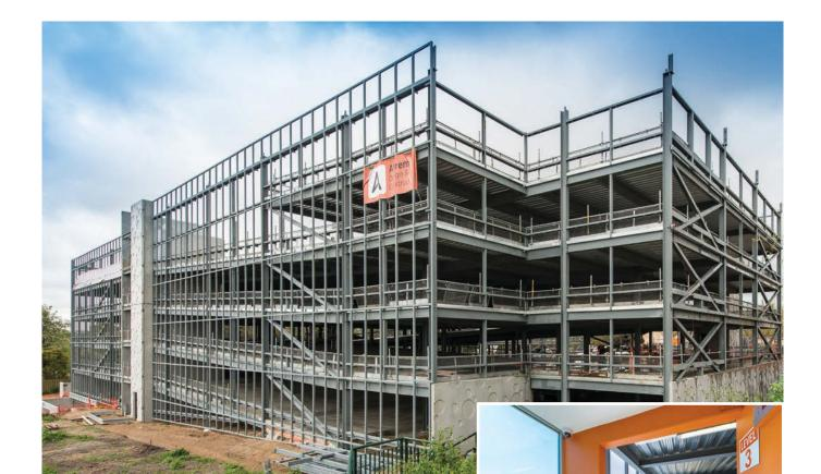
"Once primary steelwork reached level three, the next panel was erected followed by the secondary steel," he said.
