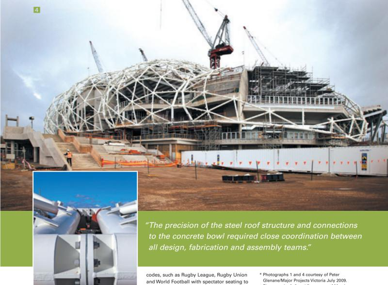
The three-dimensional nature of the roof frame also presented challenges for the structural analysis as a full 3D model needed to be built in order to represent the structure true dynamics.
