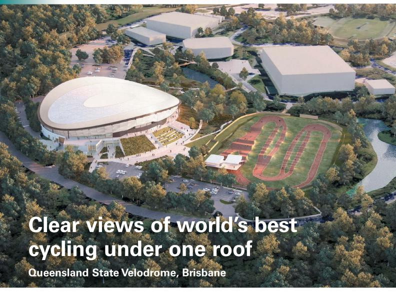
A lightweight steel frame is enabling one of the broadest clear spanning roof structures in Australia to be installed over an international standard cycling track and associated facilities for the new Queensland State Velodrome to be ready to host track cycling competition for the Gold Coast 2018 Commonwealth Games<sup>TM</sup>.
