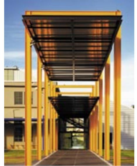
Given that external steel is exposed to continual weathering and chemical attack (hot-cold temperature cycling, UV rays, rain, hail, wind, dust, airborne chemicals such as salts from the coast and airborne acids from transportation, industrial and domestic pollution), the coating system must offer a high degree of resistance to moisture, chemicals and abrasion.
