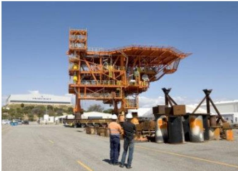
Fabricated in Australia by AGC as the main contractor, the project used 2800 tonnes of structural steel in total, with 1300 tonnes on the jacket alone, 585 tonnes in the topside section, 800 tonnes for the piles and 115 tonnes for miscellaneous installation aids.
