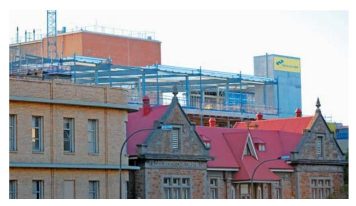
The original building was designed to the original Australian Earthquake Code AS2121 and the new extension required that the whole building be assessed against the current code AS1170.4.
