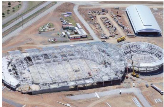
Specifically, the largest member sizes (generally Grade 450) were column legs at 200x200x8.0 SHS, while the majority of the project's 60m main arena roof truss top and bottom chords were made up of 150x150x6.0 SHS and 125x125x4.0 SHS respectively. The 42m dome selling centre comprised majority top chord members of 125x125x4.0 SHS and bottom chord 100x100x3.0 SHS, and the 6 x stable buildings majority top chords 125x125x5.0 SHS and bottoms 100x100x6.0 SHS.
