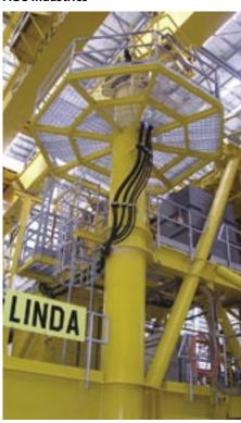
The scope of this project was for the design, supply, delivery and commissioning of the Linda Development Off-shore Gas Platform for Apache Energy on behalf of the Harriet Joint Venture. The Linda Platform stands in approximately 40 metres of ocean and is used to extract natural gas off-shore from Varanus Island. The gas is then pumped to shore via a sub-sea pipeline.
