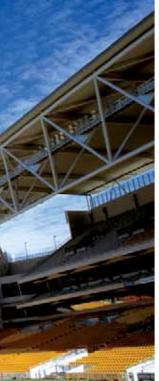
The LRJV site team implemented what they called the new 'up and under' roof construction technique for the massive new grandstands. The purlins and soffit linings were assembled in panels on the ground (under), them each section was lifted by crane into position (up).
