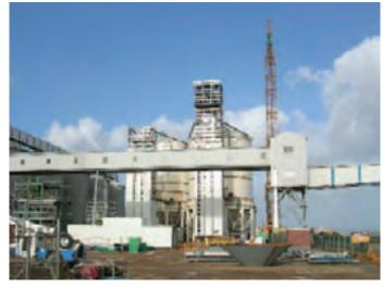
"The configuration of the new silos at the Albany port includes an under cell conveyor system. Using steel in this instance gives us more flexibility in supporting the above ground silos," Anderson added.
