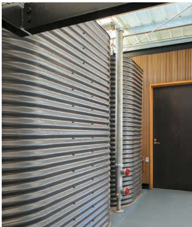
Tanks made from COLORBOND® steel in the colour Monument® collect and store water from the roof.
