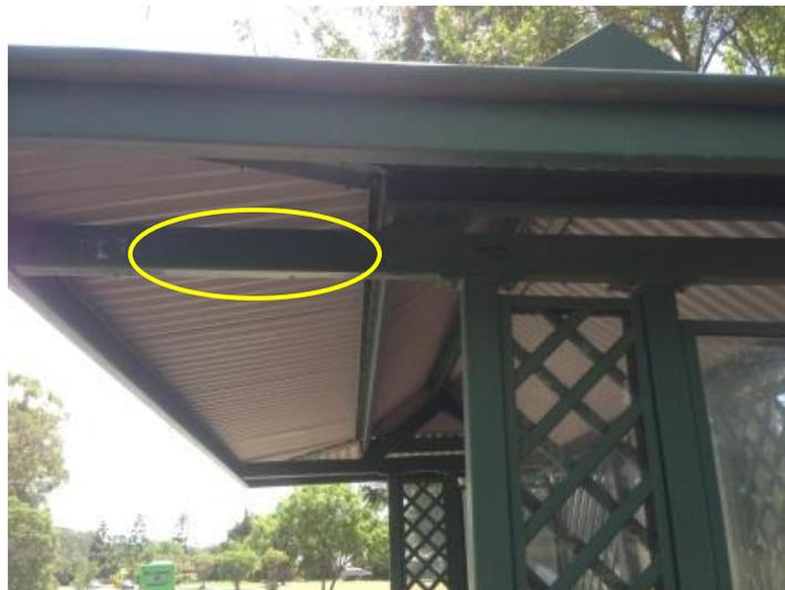
Figure 4 Example test surface (circled) suitable for chloride deposition rate testing via the Bresle method.
