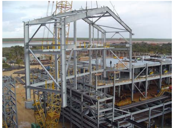
Many of the framing sections were preassembled on the ground prior to being lifted into position
