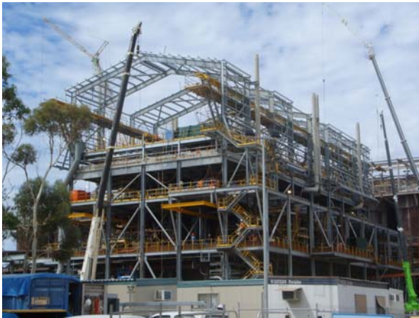
The project utilised 1350 tonnes of mainly heavy steelwork
