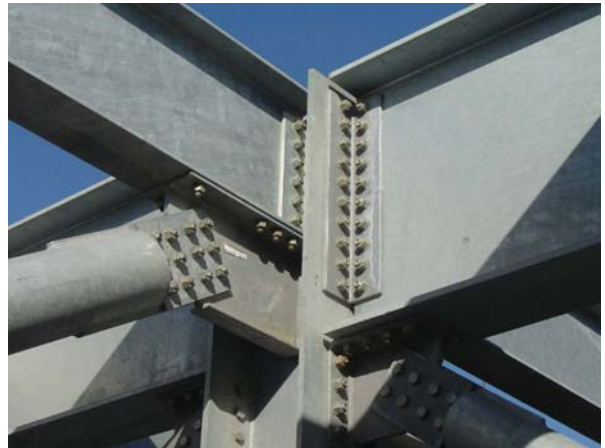
Clip angle beam connections were utilised extensively
