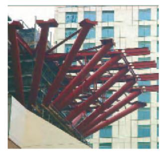
The Civic Tower under construction in the Sydney CBD takes its name from the spectacular 24-storey cantilevered tower which rises like a missile from the solid structure of the old Masonic Centre below.
