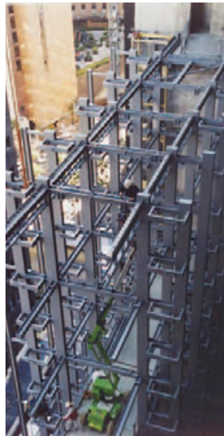
The atrium steelwork has a simplicity suited for the job. The engineers designed the atrium from basically one single off-the-shelf profile for the main structural element.
