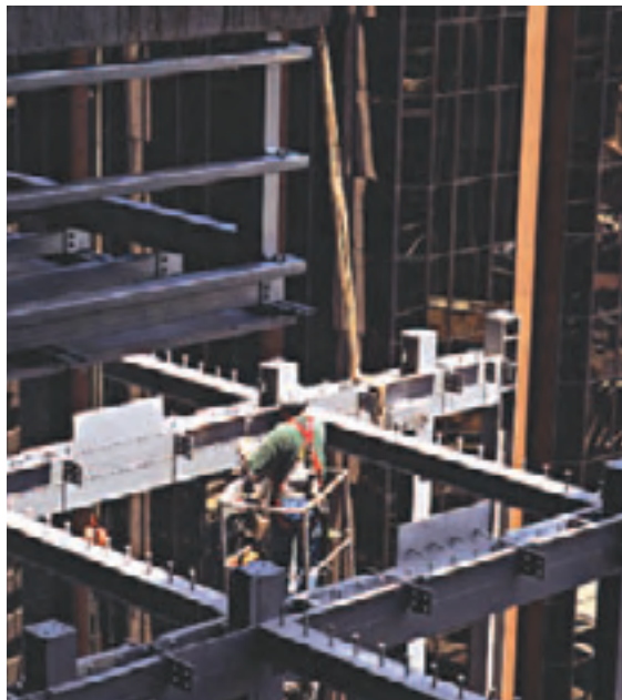
The atrium steelwork has a simplicity suited for the job. The engineers designed the atrium from basically one single off-the-shelf profile for the main structural element.
