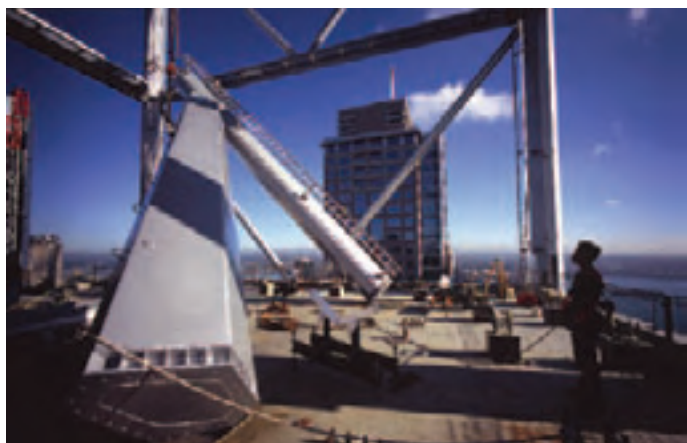
The architectural roof structure was broken into a number of repeating modules for ease of transportation and erection. Lifting lugs can be seen on the left of this section. Bovis Lend Lease site designed a program to transport, lift and connect the very large steel sections to minimise handling damage.
