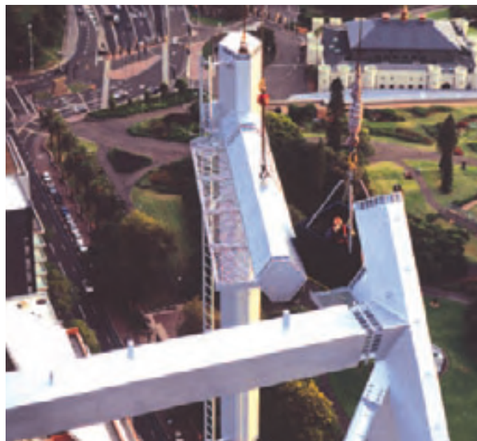
Steelworker in the "man box" high above the city. Connections from the joints to the straight members use recessed end plates and high strength tension bolts.
