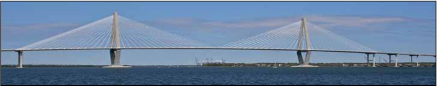
The Arthur Ravenel, Jr. Bridge (source: Wikipedia)
