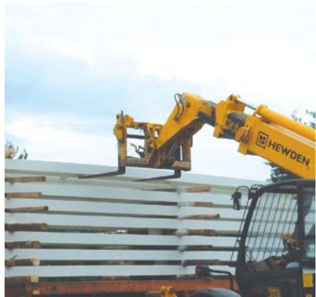
Offloading with telehandler
