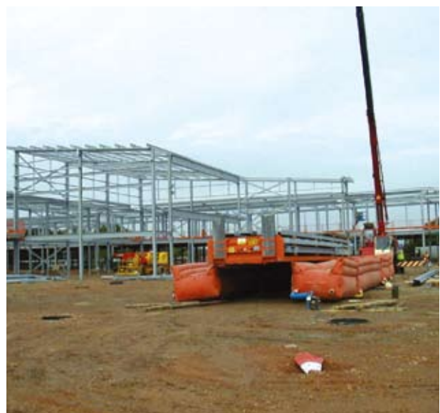
Airbags forming loading dock
