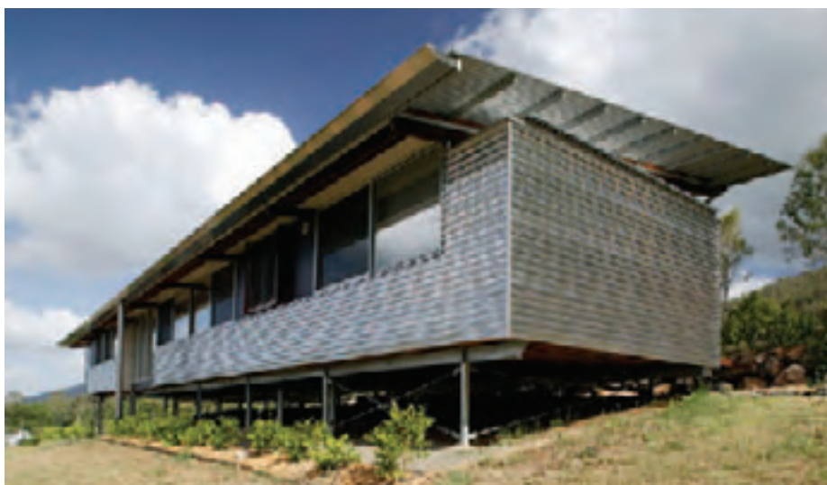
The elevated steel frame maximises the views, minimises site disturbance and provides effective low cost termite control.
