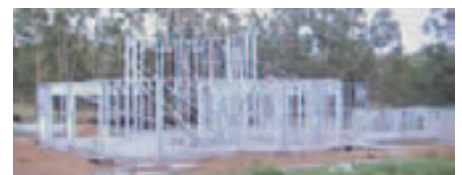
Steel frames also allow for ease of construction with pre-punched holes for installation of plumbing and electrical services.
