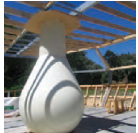
In the living room the ceiling wraps down to an internal bulb-shaped water tank.
