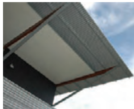
The 120 deep steel top hats, used as roof purlins were easy to install on site by carpenters. Direct fixing to the timber roof beams avoided the need for cleats and brackets.
