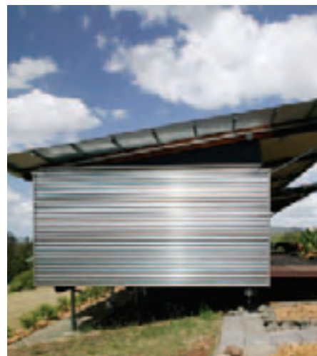
The large skillion roof creates a generous sheltered outdoor area and high internal ceilings.
