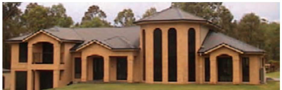
This feature combined with the use of Colorbond® roofing allowed for wide spans for the steel roof trusses thus providing an economical and durable structure.
