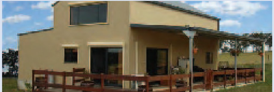
In the American style barn the mezzanine loft is also constructed from steel sections.
