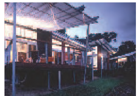
Steel framed tropical rooftops catch and direct the prevailing south easterly sea breezes through to doors and windows
