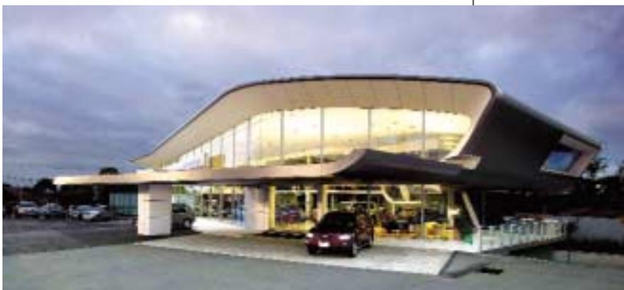
The building incorporates bare steel beams and columns throughout utilising OneSteel's **300PLUS®** range of structural sections.
