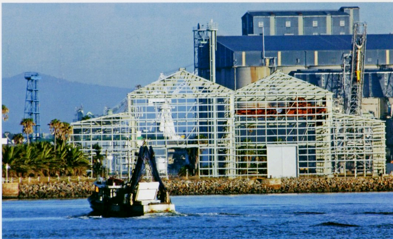
The Newcastle Dockyard building on Dyke Point in the foreground is being recycled into a luxury yacht service facility. The purlins are newly galvanized, but the 100 year-old major structural steel sections have been retained and repainted.
