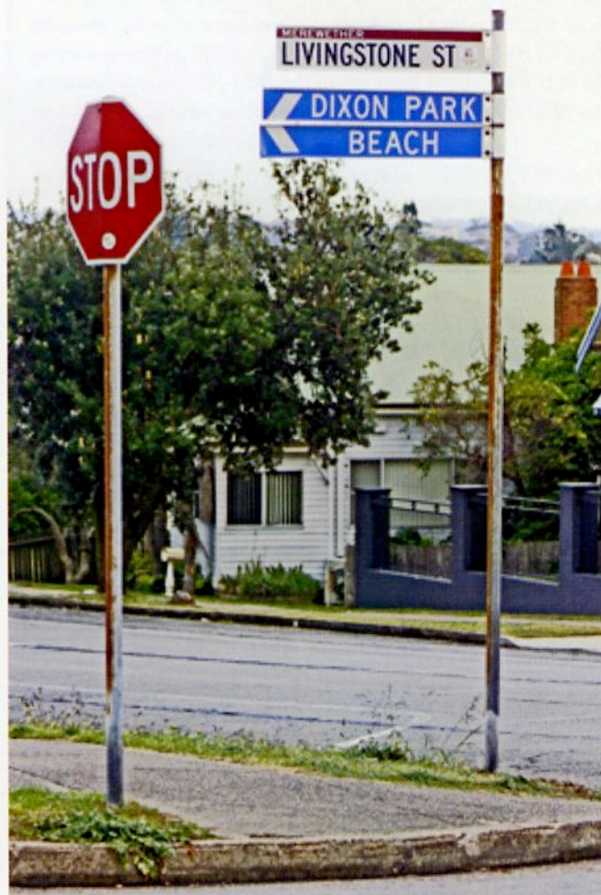
Orientation is critical in sheltered areas. These galvanized signposts show the clearly defined corrosion stress on the rusty (southerly) side of the posts facing the ocean 400 m distant.
