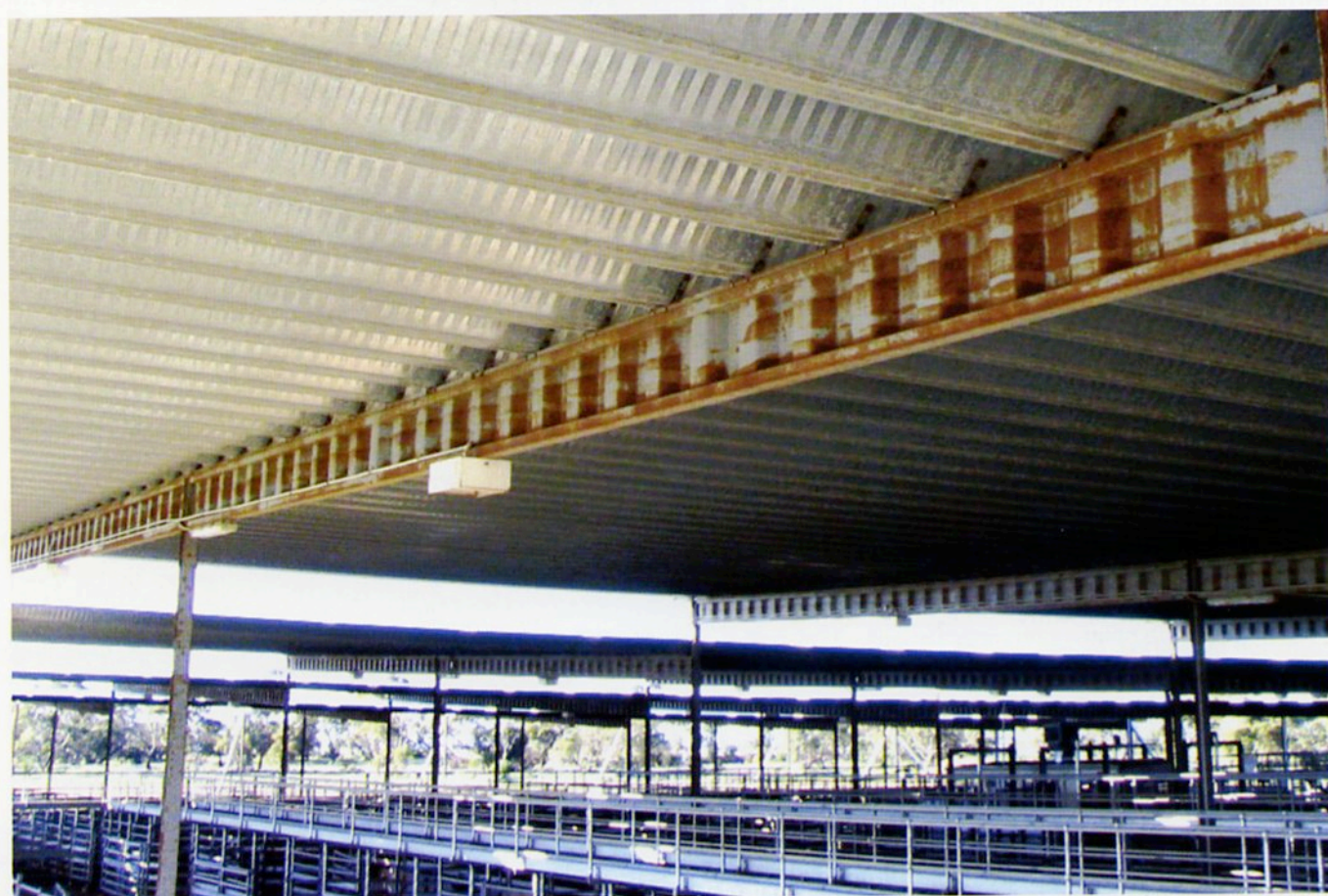
This large open roof structure located north of Adelaide SA shows the effects of chloride induced corrosion stress after 2 years on the windward (bottom) and leeward (top) sides of the main roof beams.
