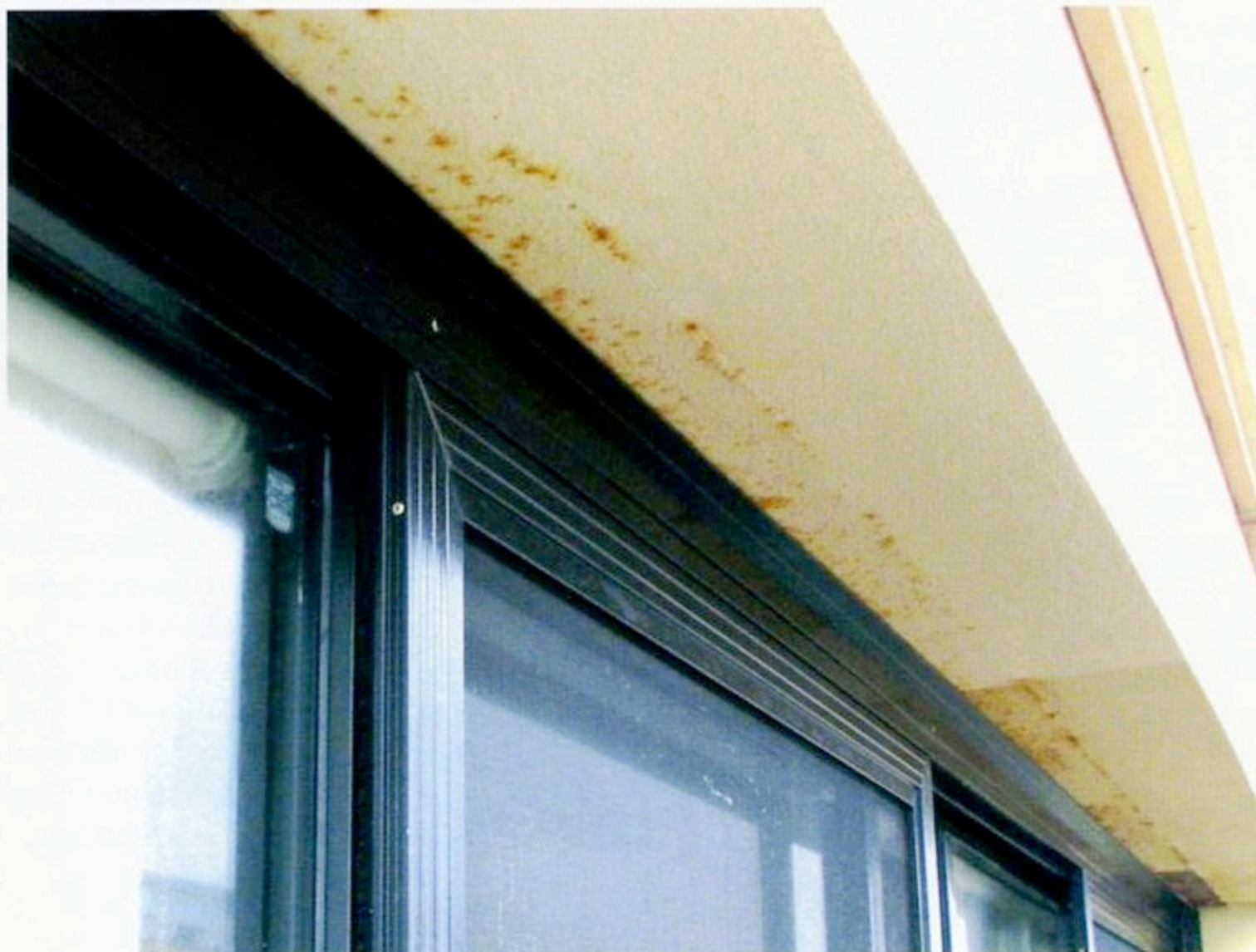
Lintels are always in sheltered locations on building facades and need to be adequately protected, unlike this 3-year old installation - Page 14
