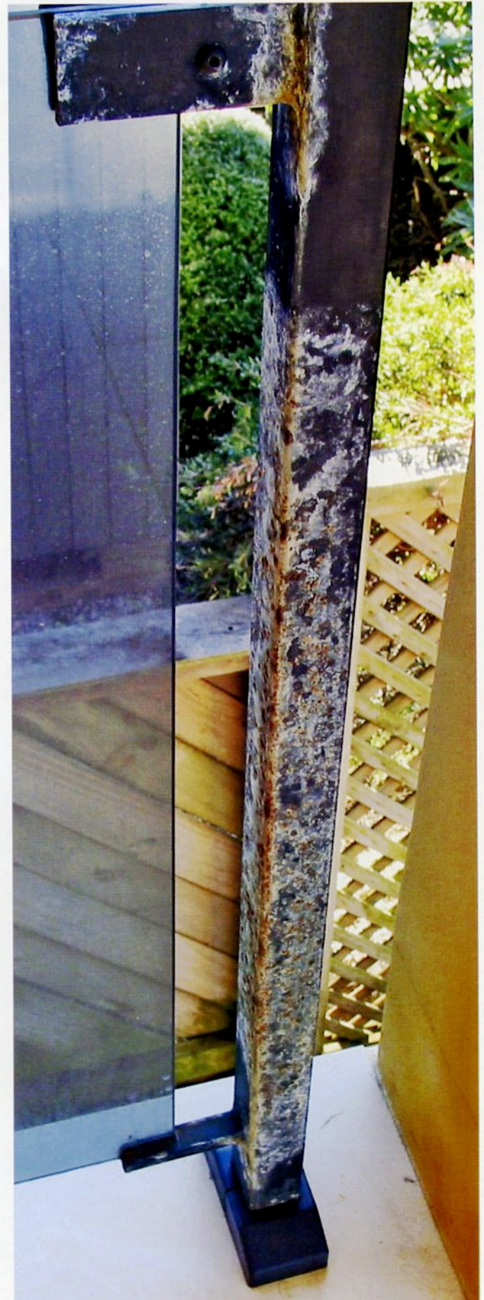
Total powder coating failure on this bayside verandah stanchion within 2 years on sheltered area of the verandah.
