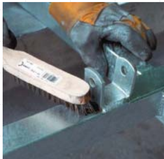
Surface to be repaired is cleaned by wire brushing.
