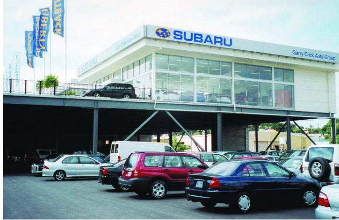
(L) A suspended slab at street level accommodates four showrooms with the service area accessed via a ramp to the lower level.
