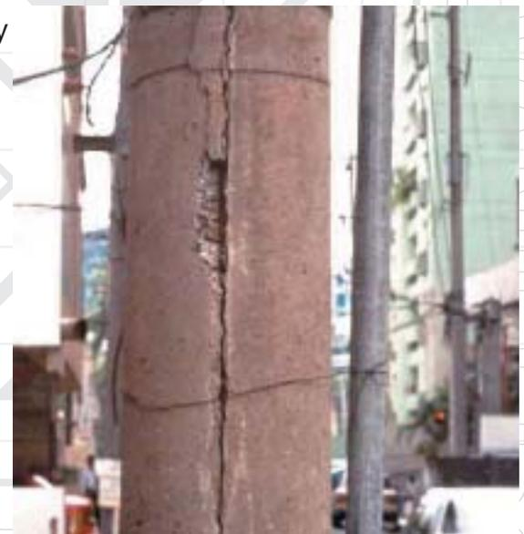
The corrosion of the steel reinforcement in this concrete power pole has caused it to split from end to end
