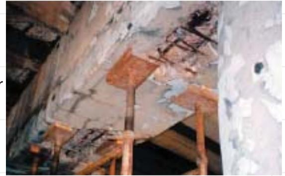
*The corrosion of the reinforcing bar in this road bridge in North America has occurred because of poor rebar placement combined with the use of de-icing salts on the road.*
