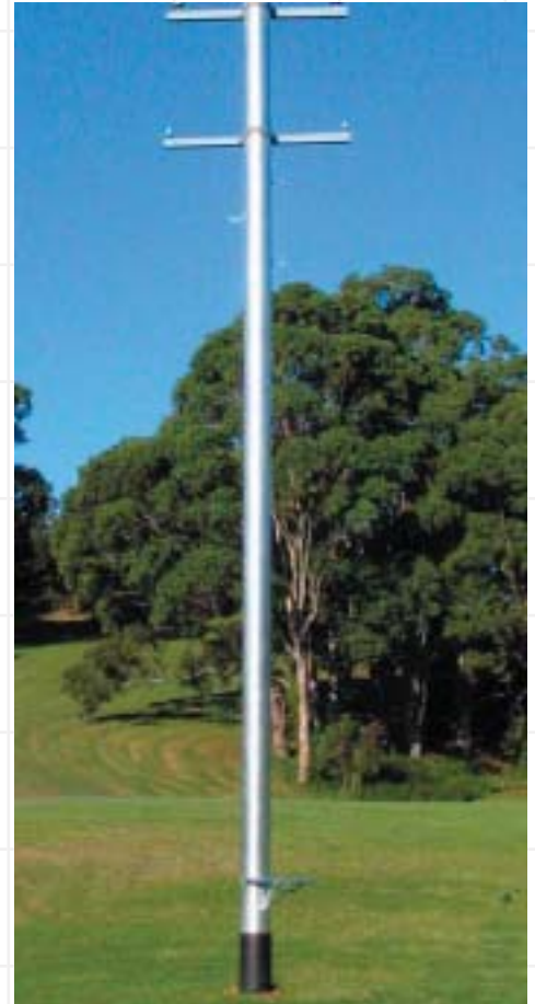
Galvanized steel poles have been direct buried for many years. BlueScope Steel's newly developed Sureline pole is designed for a minimum of 50 years in-ground service, using heavy galvanized coatings and membrane systems at the ground line.
