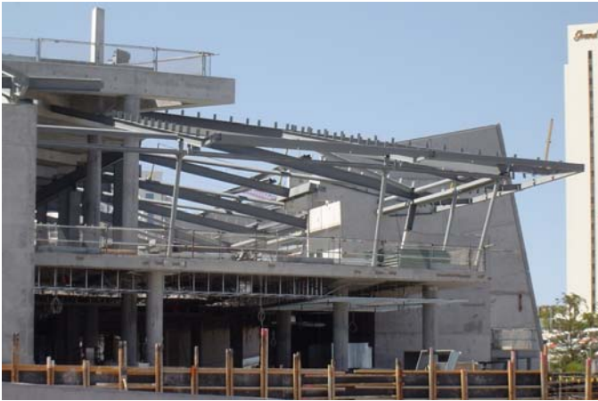
Complex connection issues were able to be resolved easily with the use of the 3D model
