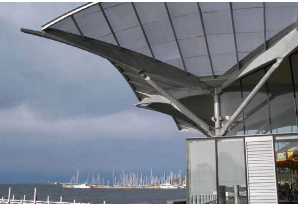
4. The galvanized coating is subject to corrosion at a predictably slow rate, between one-seventeenth and one-eightieth that of steel, depending on the environment to which it is exposed.
