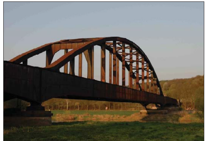
A weathered steel bridge in Höxter, Germany
