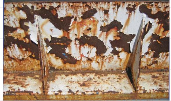
*Poor quality paint systems can accelerate steel corrosion by concentrating pollutants and corrosion cells around and under the paint film.*
