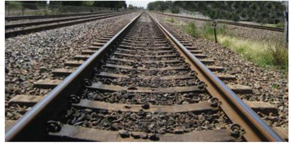
*There are many instances where steel is used without a protective coating. Rail lines are a good example and have excellent durability in most Australian environments.*
