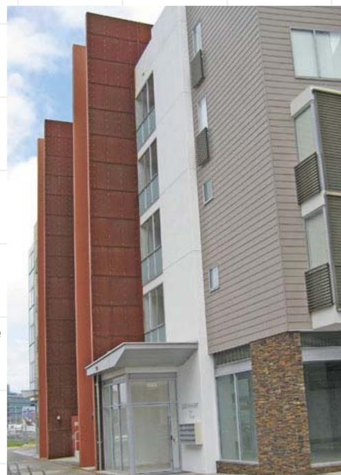
*These architectural elements on a harbour-side building in Newcastle, NSW are fabricated from uncoated weathering steel.*
