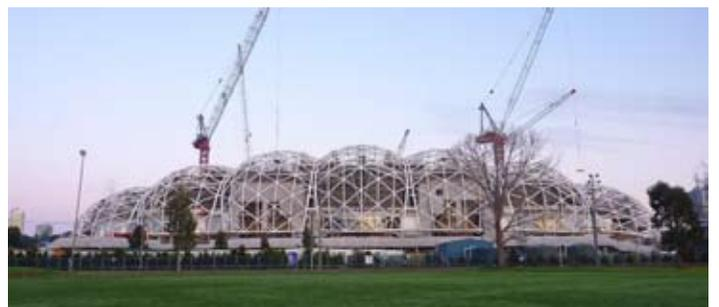
fabricators, therefore reducing fabrication and overall construction time. The design also provided some repetition to simplify the construction process. Each of the four quadrants is symmetrical, allowing repetition of cladding panel shapes and sizes.
