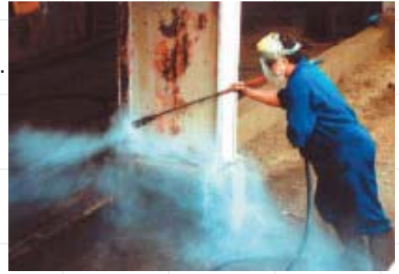
Ultra-high pressure (35,000 psi+) water blasting is an effective way of preparing contaminated surfaces for maintenance painting, particularly where chlorides are present.
