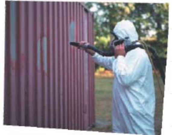
Special abrasives such as Sponge Jet media can be used for delicate removal operations
