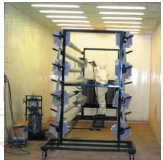
Large galvanized fabrications such as these lighting poles are garnet blasted prior to powder coating. This improves the powder coating adhesion and ensured that the zinc surface is free of oxidation products.
