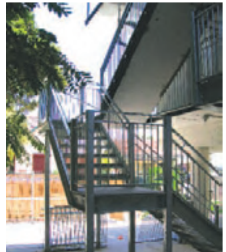
The new enclosed steel stairway.
