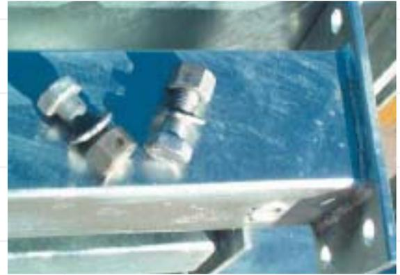
*Galvanized bolts require their nuts to be tapped oversize to allow clearance for the galvanized coating on the thread. Galvanized nuts are not galvanized internally and rely in contact with the coating on the bolt for their corrosion resistance.*
