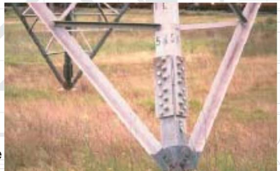
*Bolted connections on electrical transmission towers have their own standard for bolts in these critical galvanized structures.*
