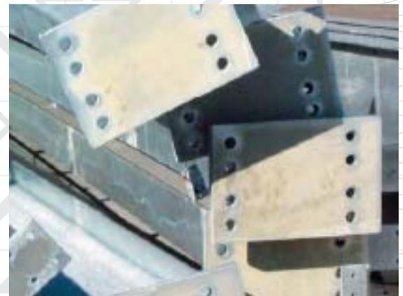
*Where the hot dip galvanizing process generates gray coloured coatings, the surfaces are deemed to comply with the 0.35 coefficient of friction minimum requirement for friction grip bolted connections.*
