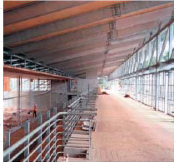
*The Sydney Olympic Shooting Centre is an excellent example of a significant bolted galvanized structure where fast erection and low long-term maintenance were a requirement of the design.*
