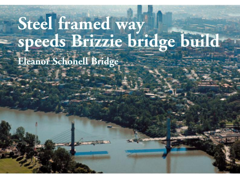
Design and Construct Lead Contractor, John Holland selected a steel framed deck for the main and back spans supported by steel cable stays for a new bridge for busy Brisbane as this approach produced a lighter structure requiring less support.
