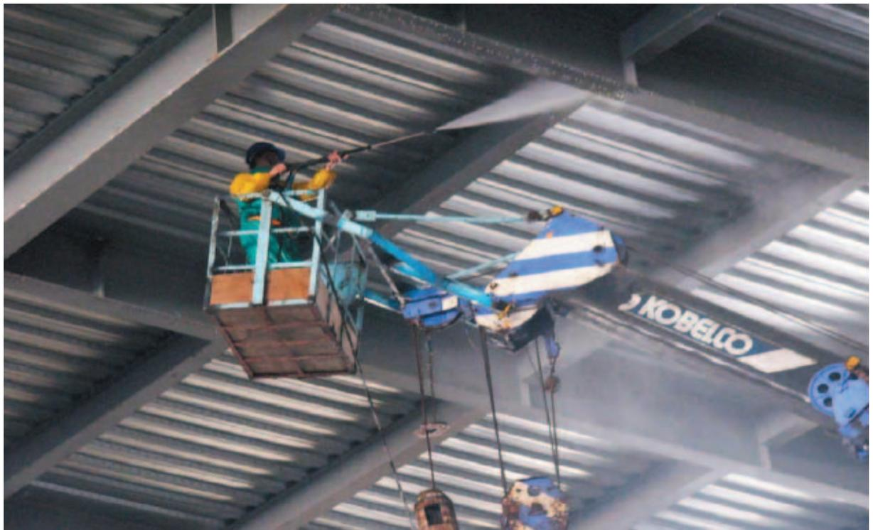
**Figure 10: Intumescent paint being applied in the field**
