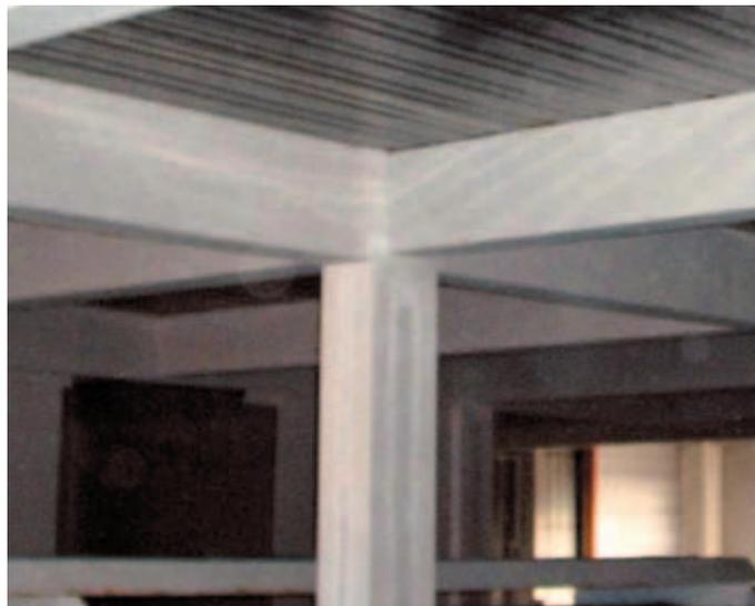
**Figure 7 and 8: Steel sections clad in fire proofing board materials**
