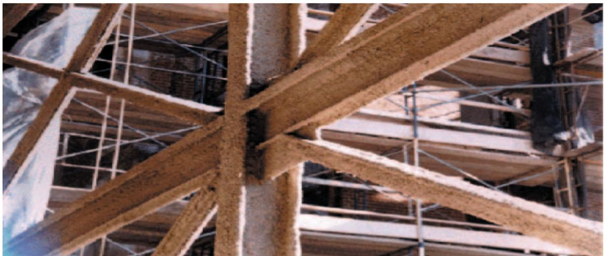
**Figure 5: Conventional spray applied fire protection material**
