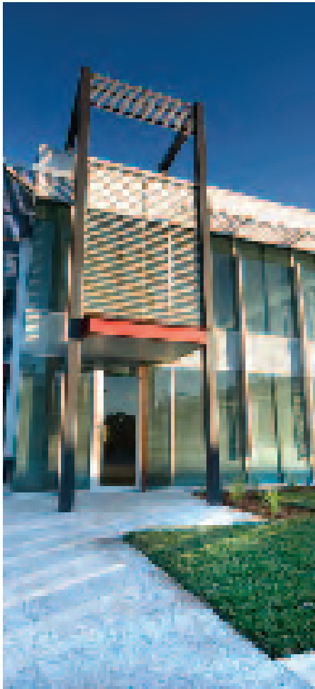
The combination of glass curtain walls, Alucabond and precast concrete gives the facades a modern look.
