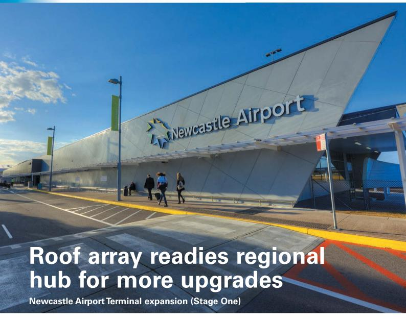
A well targeted lightweight steelwork package has capped off the partial redevelopment of a busy airport terminal located at the regional centre servicing the Hunter in NSW, ready to be extended further when required.
