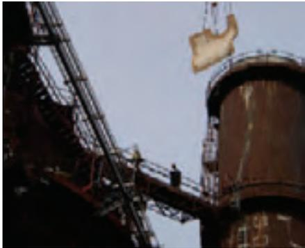
The steel was blasted and coated then craned into position for final fabrication before installation 40 metres above the base of the blast furnace.
