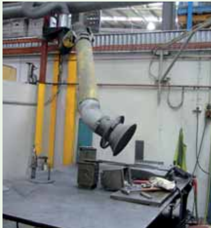
Fixed extraction unit assists in removing exposure to fumes, the unit is manoeuvrable to ensure fumes are taken away from the welder at all times.
