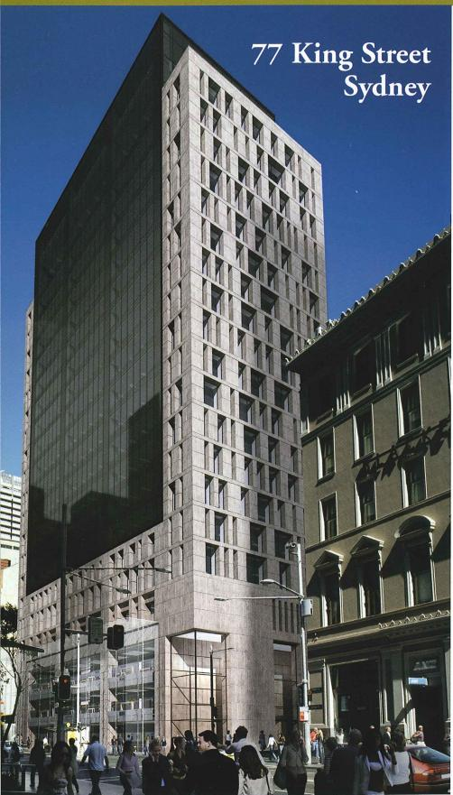
An established inner-city building has received a new lease of life with a lighter-weight composite steel frame solution providing five new levels (four floors and steel roof) that allows more advanced, roomier and environmentally friendly facilities.
