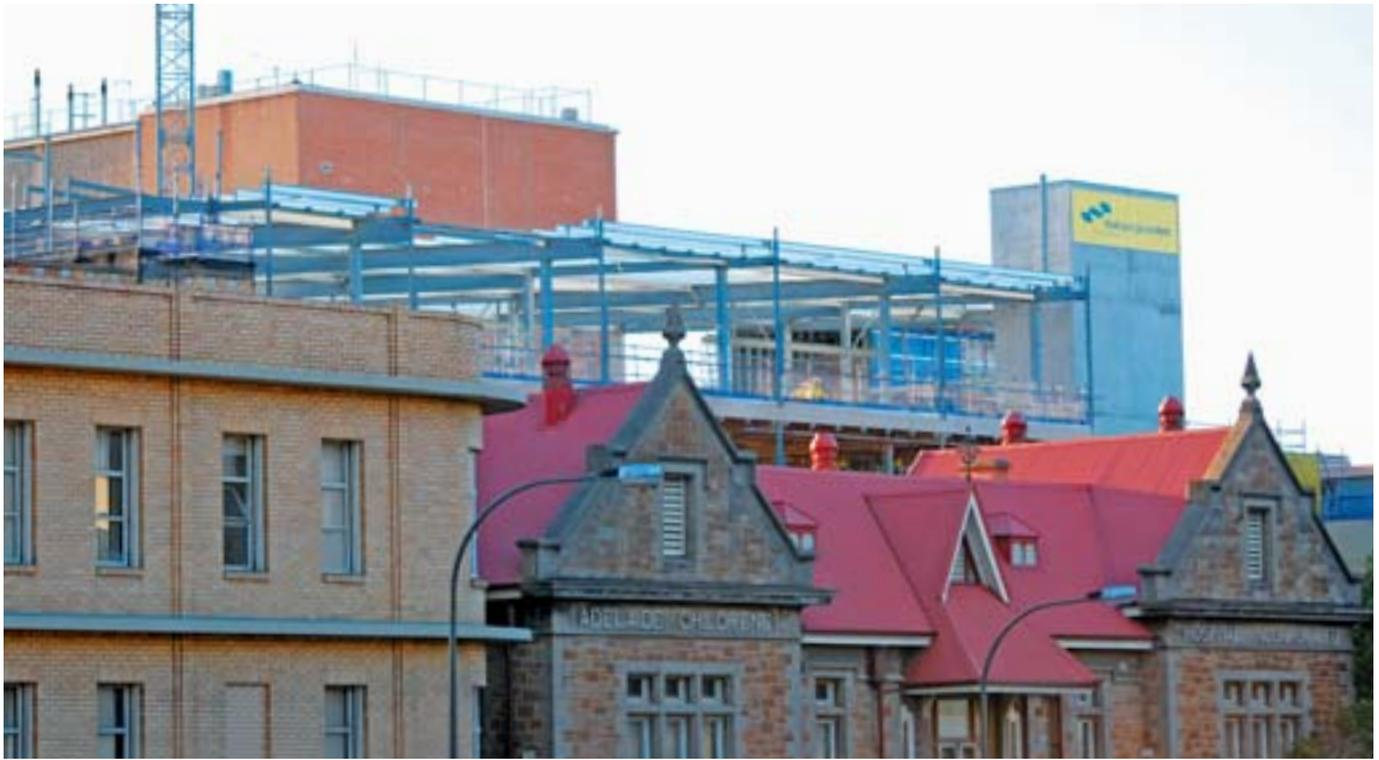
The original building was designed to the original Australian Earthquake Code AS2121 and the new extension required that the whole building be assessed against the current code AS1170.4.
