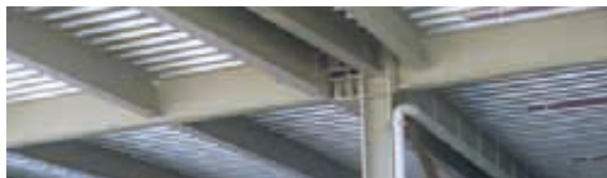
Figure 5.8 Corbel expansion / contraction joint.
