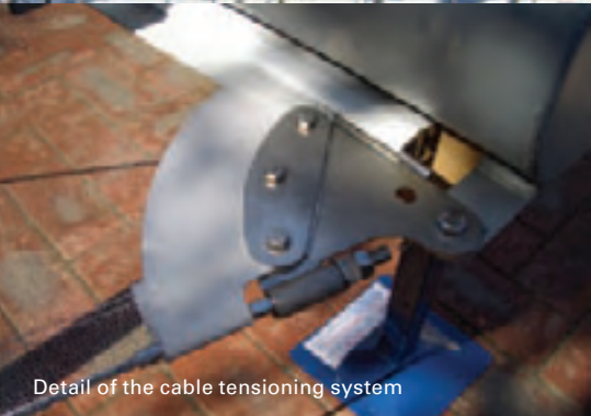
Typical footing detail, located at the base of each arch
