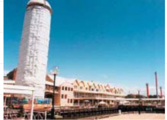
The maintenance painting of structures in public or environmentally sensitive areas required costly containment systems to meet EPA requirement. The cost of repainting this tourist observation tower in Newcastle, NSW exceeded its initial installation cost after only 12 years.
